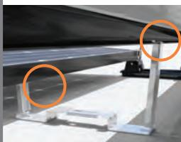
Press the Upper and Lower Mid-Supports onto the module frame.
